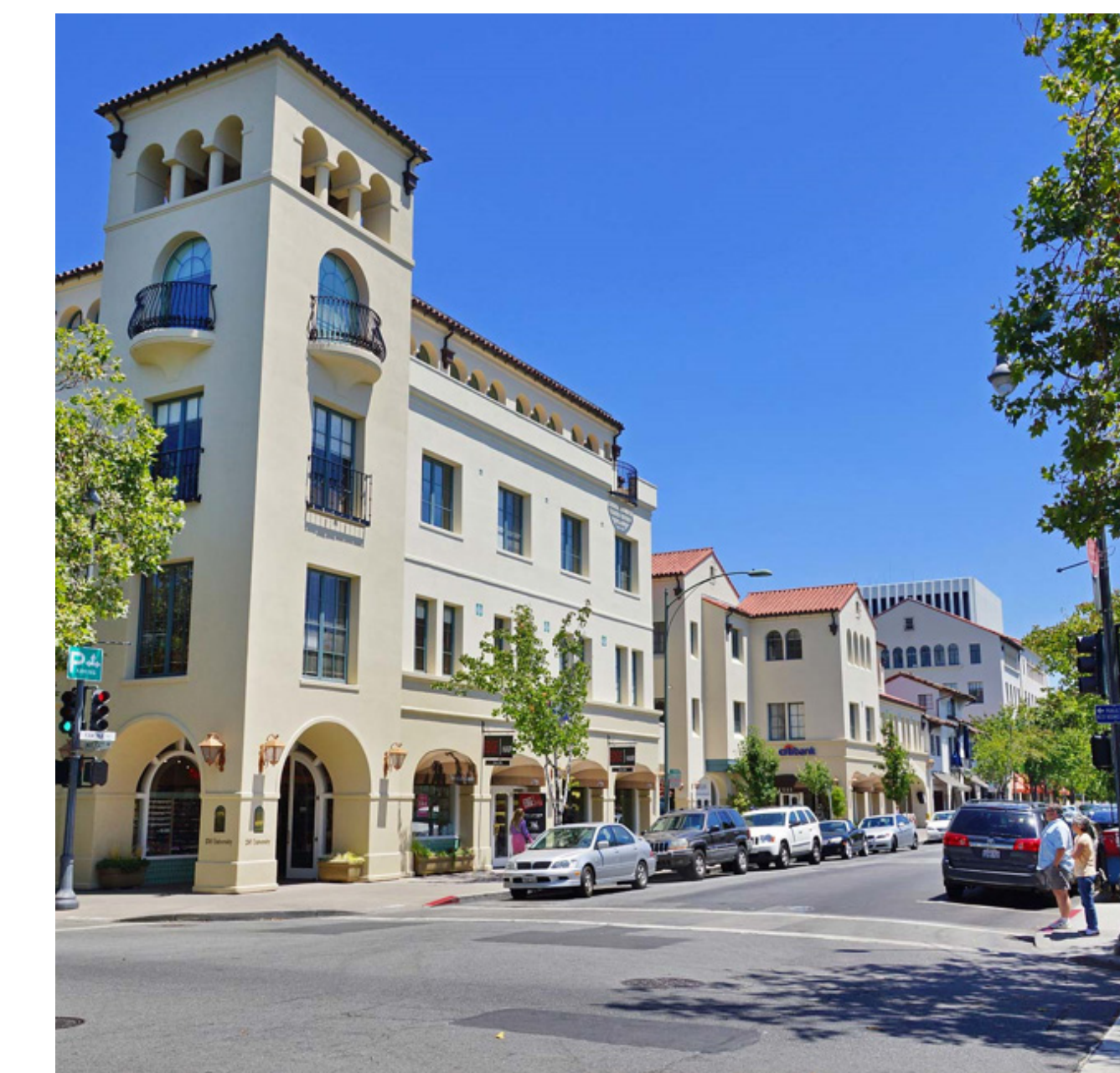
Downtown Palo Alto, CA Height: 55 ft (not including tower) Floors: 4 Strategy: Tower and stepped back height at top
