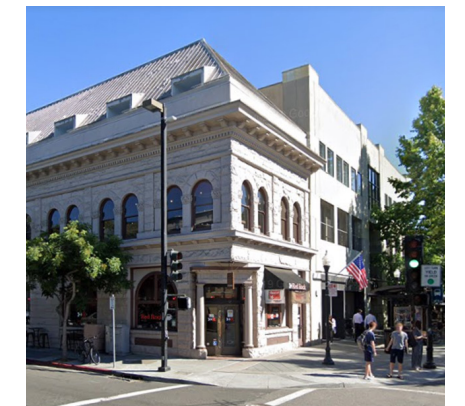
Downtown Mountain View, CA Height: 45 ft Floors: 3 Strategy: Varied facade and shape
