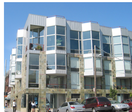
Variation in building face
